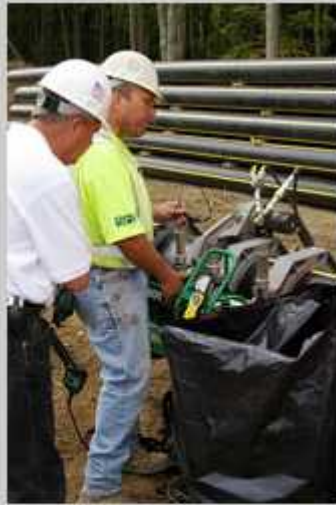
The 12-inch SDR 9 is faced off in a TracStar 412. Photo courtesy of R.H. White
